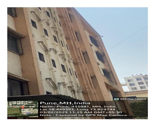
Rain water collected from building terrace and through underground gutter collected in open well
