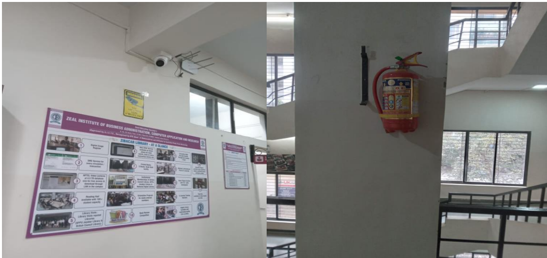
Safety Measures : Fire Extinguisher and CCTV
