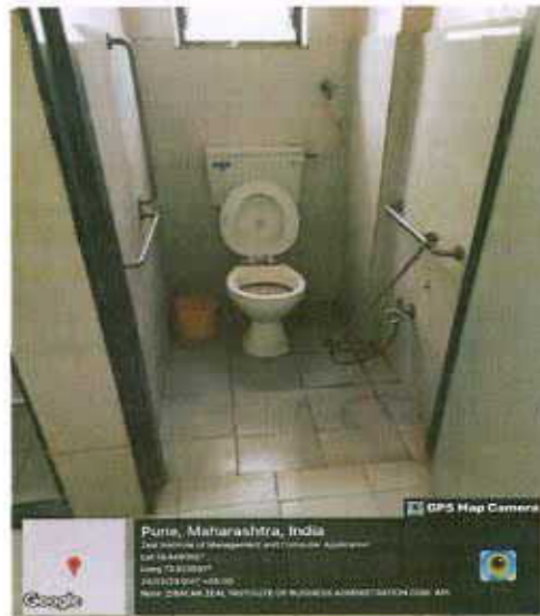
Photograph showing Divyangjan Washroom.
