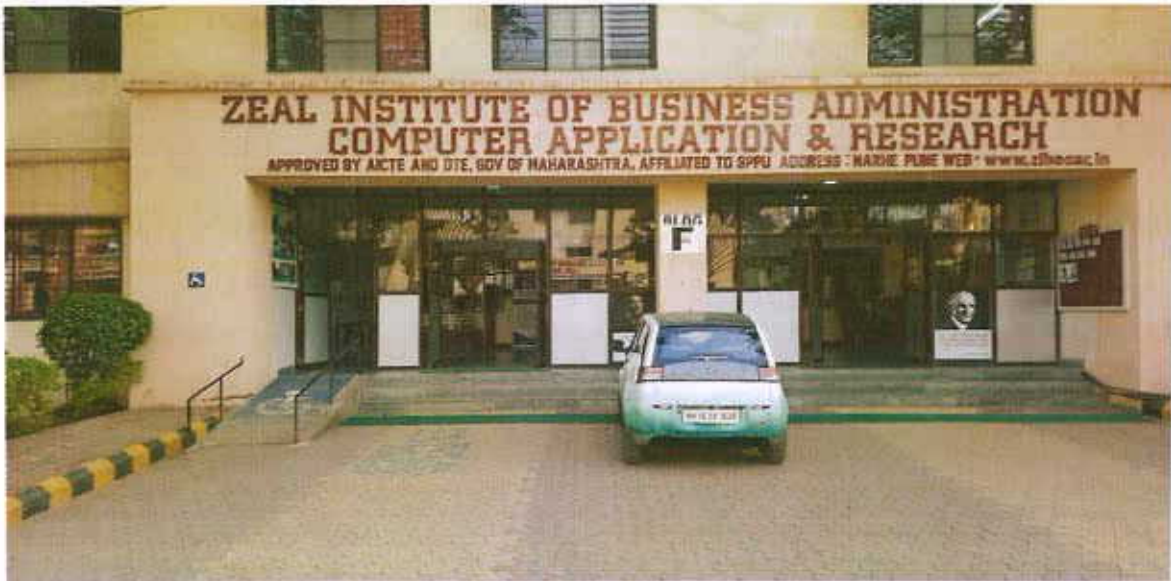
Photograph showing Divyangjan Ramp and Parking area.
