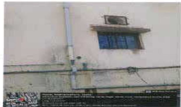
Photograph showing open well recharge through rainwater harvesting
