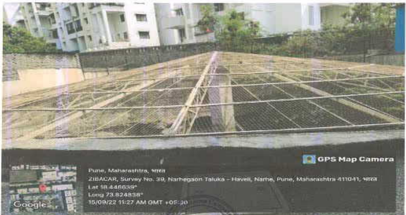
Photograph showing open well recharge through rainwater harvesting
