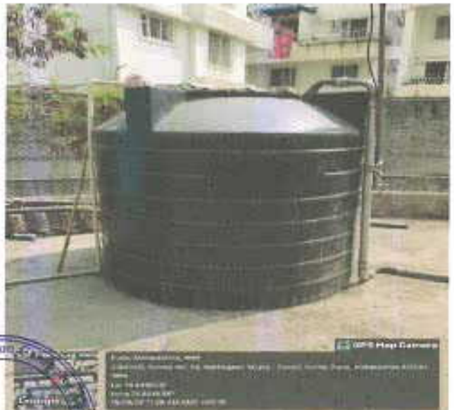
Rainwater is collected in the reservoir through Pipes
