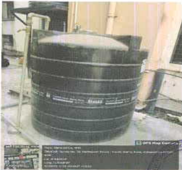
Rainwater is collected in the reservoir through Pipes
