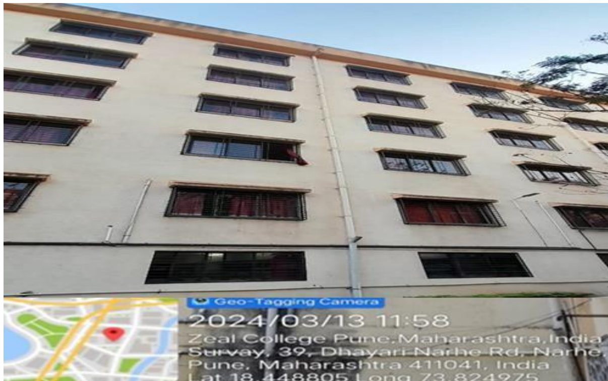
Image-7.1.4 (1a) -Rain Water Harvesting System
