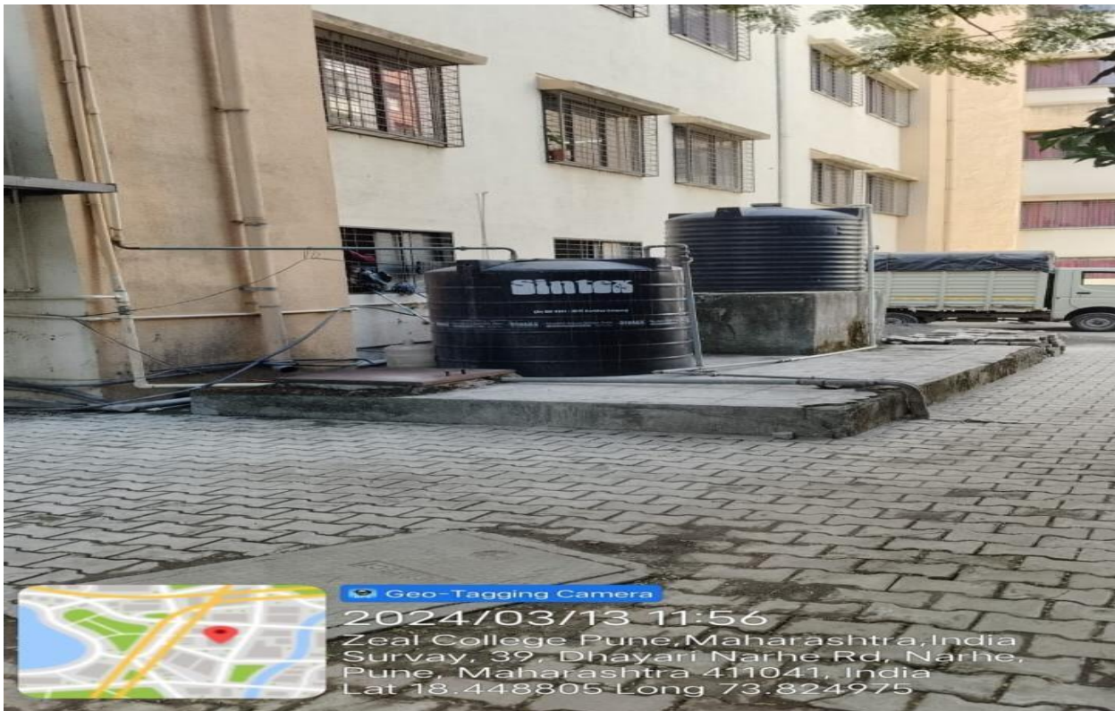
Image-7.1.4 (3A) - Construction of tanks and bunds @ ZES Campus
