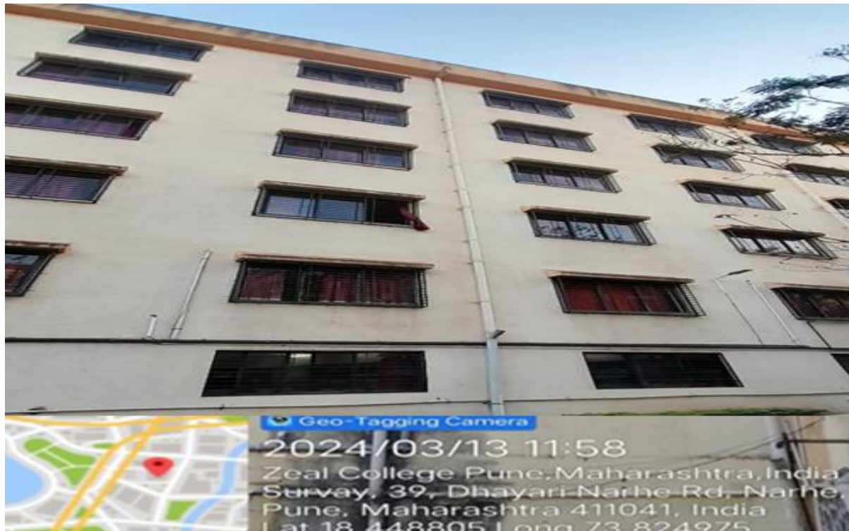
Image-7.1.4 (1a) -Rain Water Harvesting System
