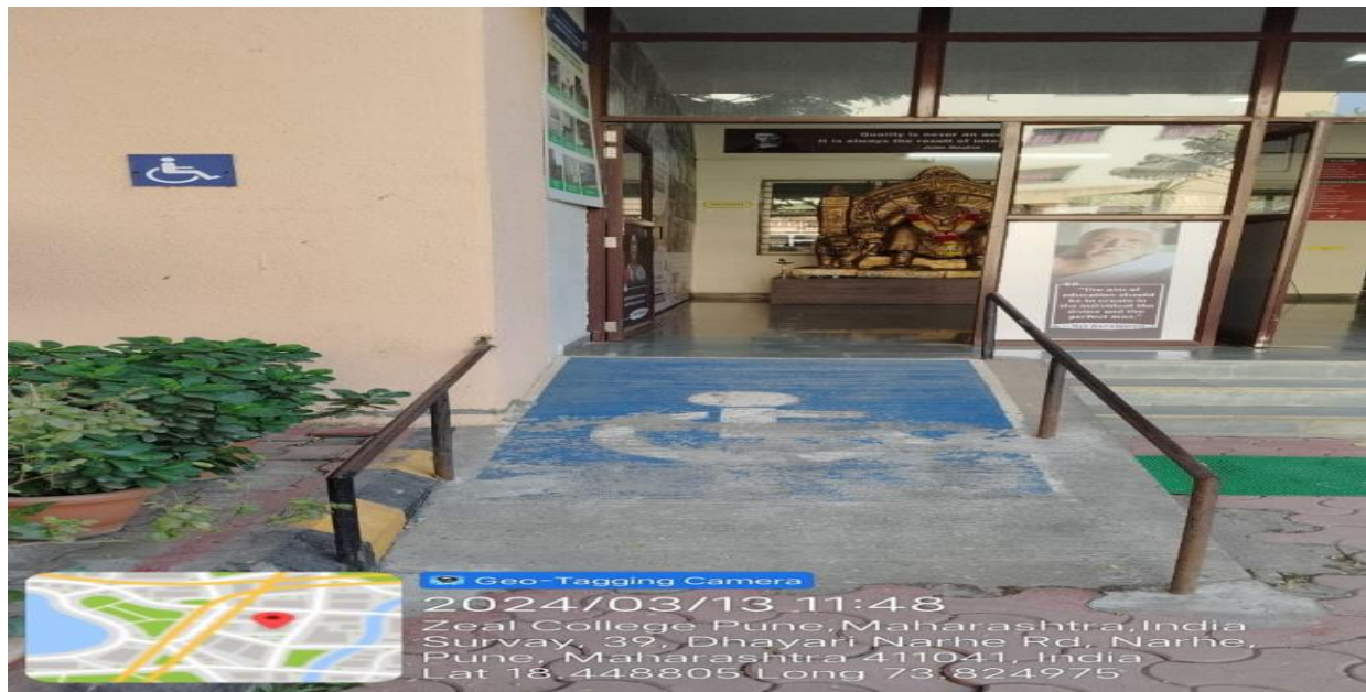
Image-7.1.7.1-Ramp for ease of access at entry point ZIBACAR
